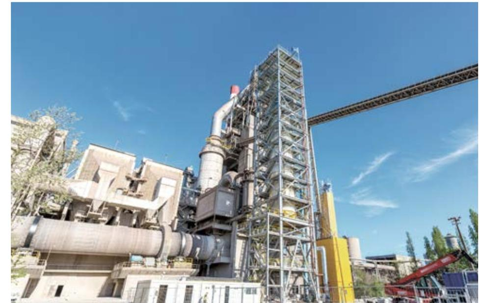
At the HeidelbergCement plant in Lixhe, Belgium, the LEILAC consortium is working on capturing CO<sub>2</sub> in its purest form, thereby reducing the ecological footprint of cement production.
